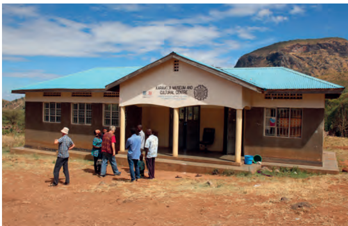
Abb. 1 Karamoja Museum and Cultural Centre, Aussenansicht
